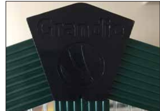
Exterior view of mid roof cap JG01.
