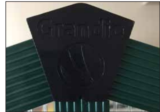
Exterior view of mid roof cap JG01.
