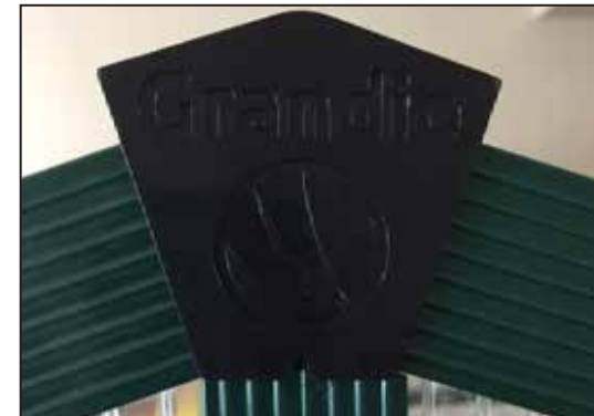
Exterior view of mid roof cap JG01.
